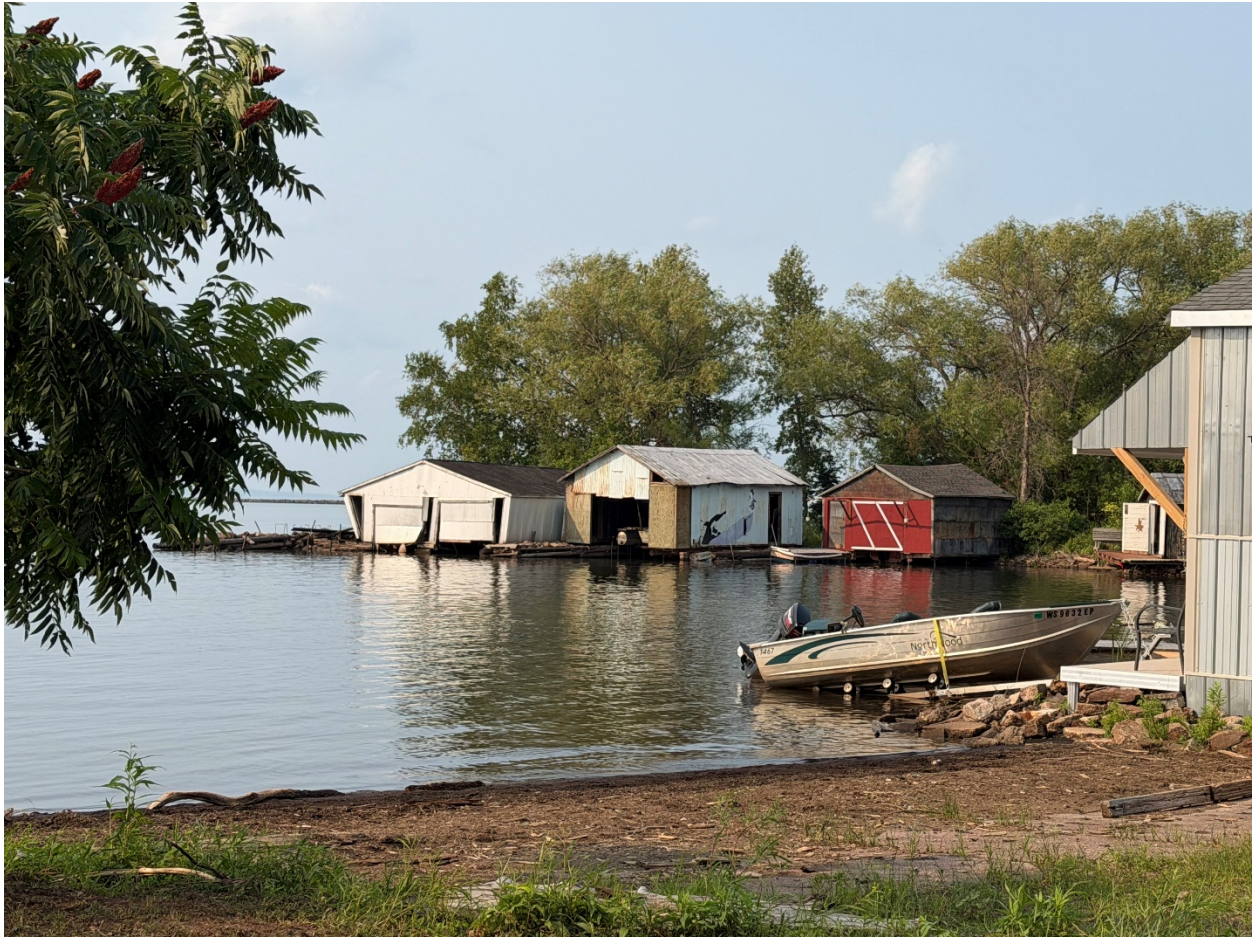
Existing condition of boat houses to North/East
