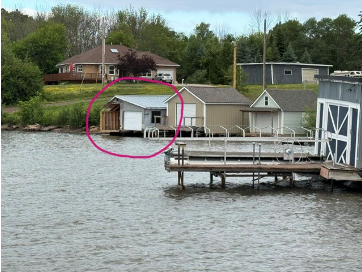
View from water – window can be seen on west side
