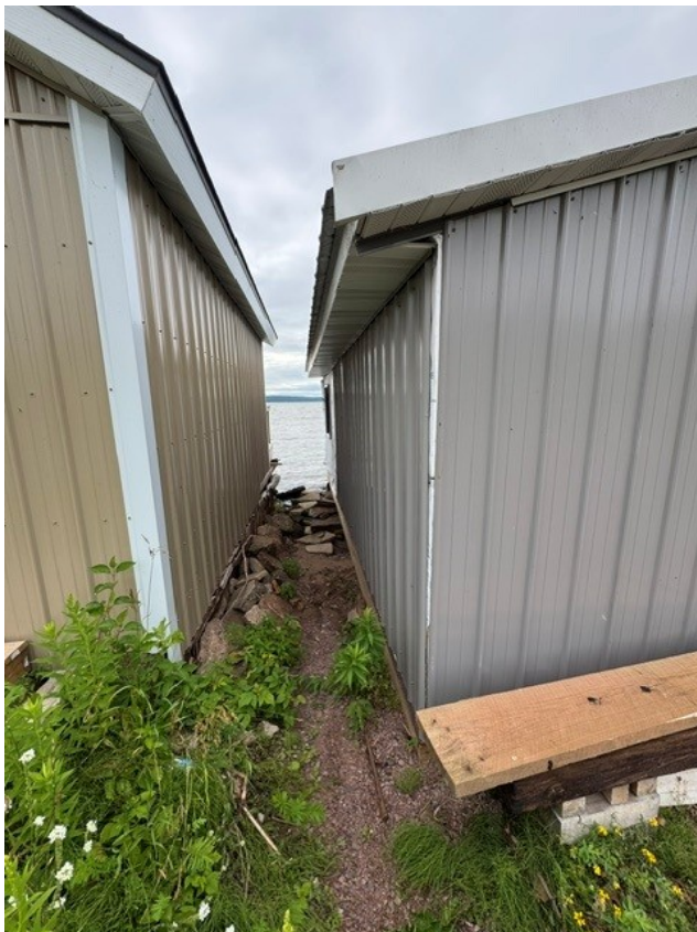
Proximity to adjacent boat house installed window on north end can be seen
