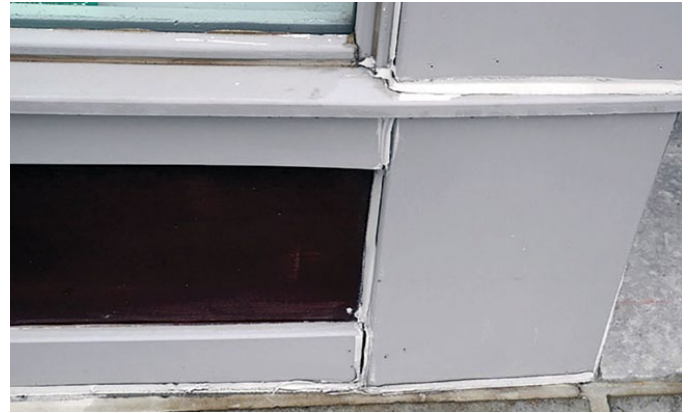
Figure 12. Cellulose composite materials, like wood, expand and contract with moisture. Here it was used to reconstruct a missing storefront. Unlike solid wood that is dimensionally stable parallel to the grain, this composite moves equally in all dimensions, resulting in gaps that were not adequately anticipated in the design. Photo: John Sandor, NPS.
