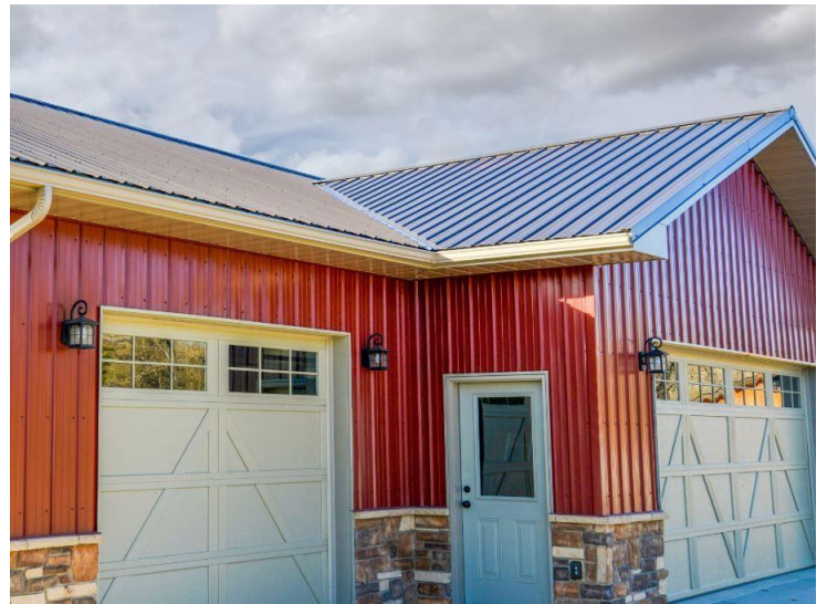
Brightly colored ribbed sheet metal roof with exposed fasteners. This would not be desirable within the city.
