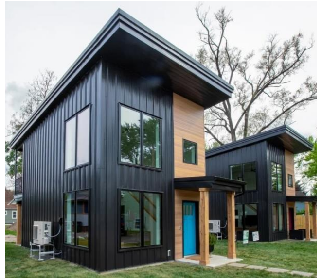
Painted ribbed sheet metal with exposed fasteners. The difference in quality and finish of material is evident with gauge and finish.
