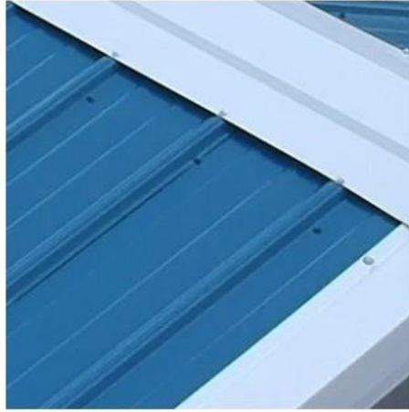
ribbed sheet metal roof
