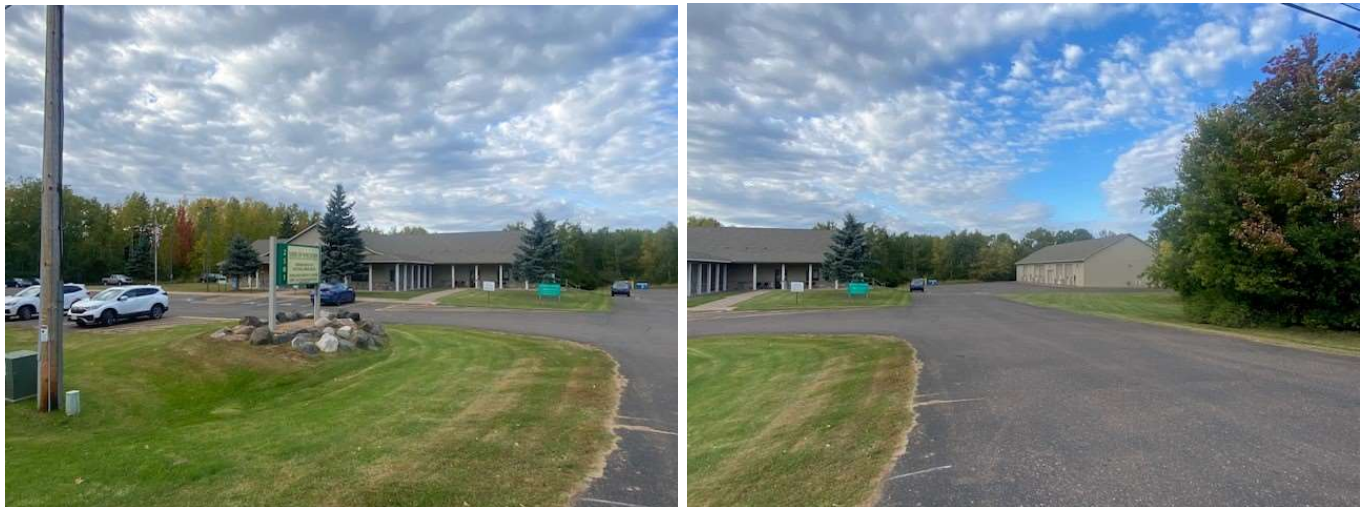
These images show the entry view from Golf Course Road to the site. In the left photo is the primary building containing the DMV and DNR offices with the lighted parking lot out front. In the right photo is the driveway leading to the existing storage building to the rear of the property.
