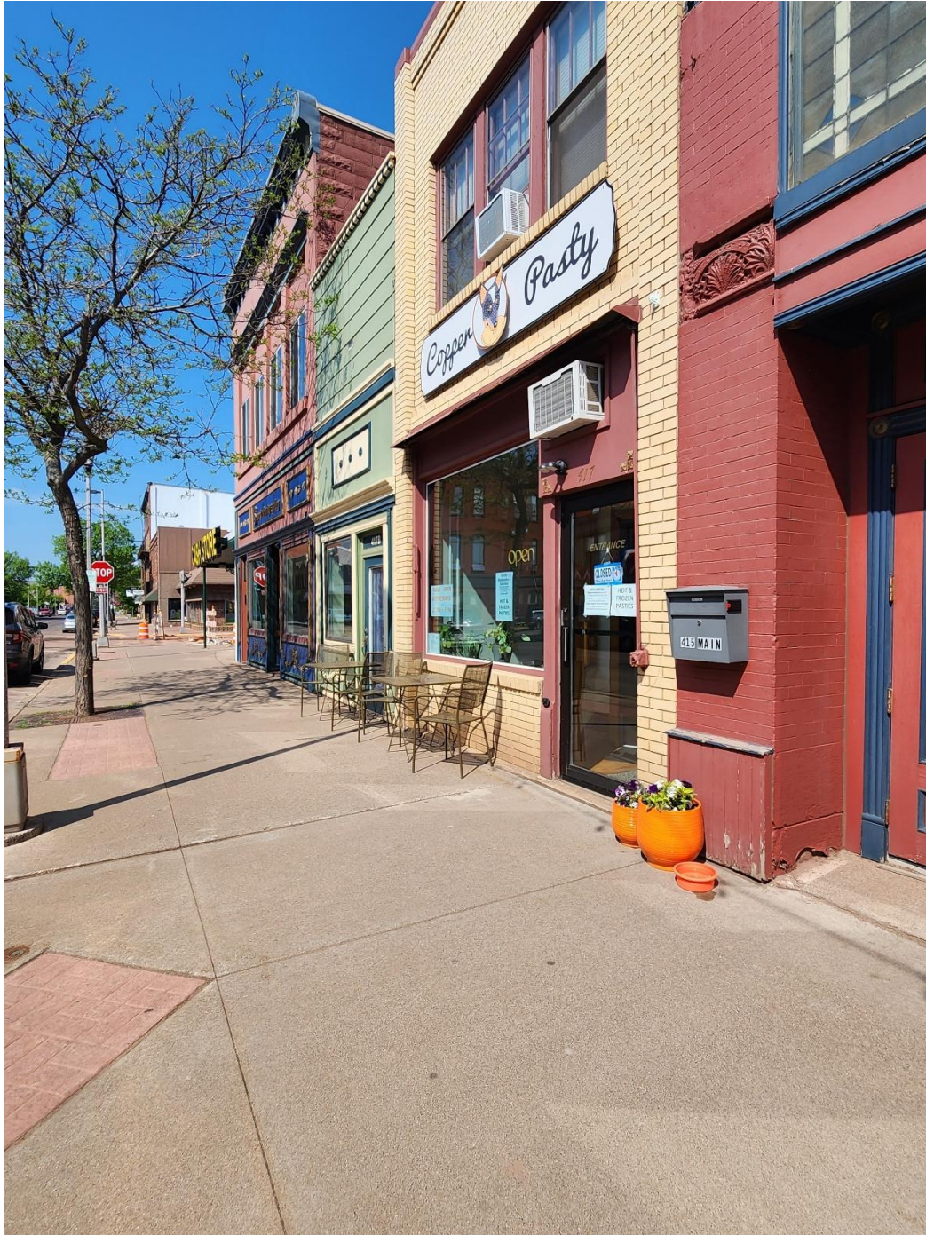
Exterior view of building facing West – clearer view of tree that obstructs view coming from the West toward East Main Street.
