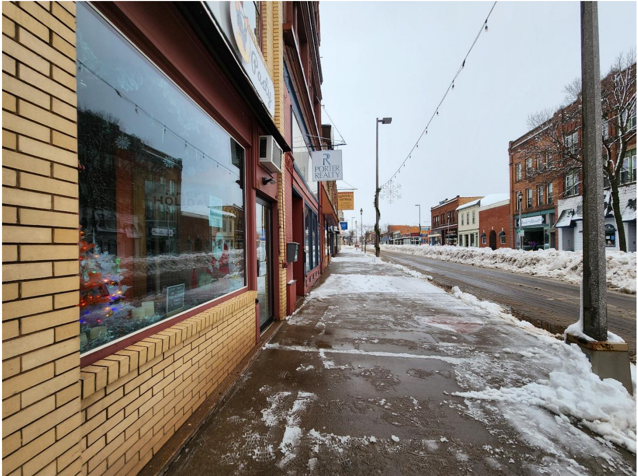
View of neighboring protecting signs.
