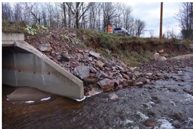
Delfield Road, Town of Ashland, is highly vulnerable to upstream headwater incision, landslides, and excess deposition. Photo: WI Wetlands Association
