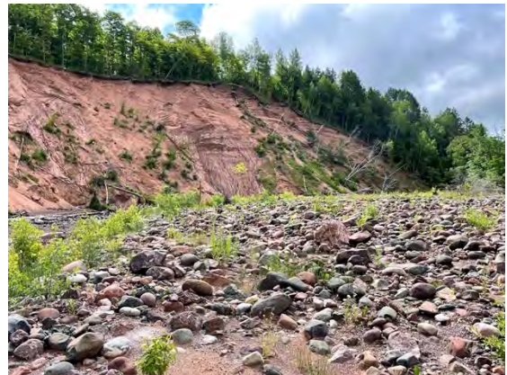
Excess sediment and debris from a 2016 flood-related bluff failure buried floodplain wetlands. Photo: WI Wetlands Association
