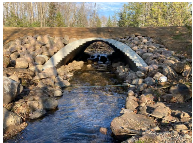
A climate resilient road-stream crossing created on a town road, designed with the USFS Stream Simulation Methodology. Photo: Trout Unlimited
