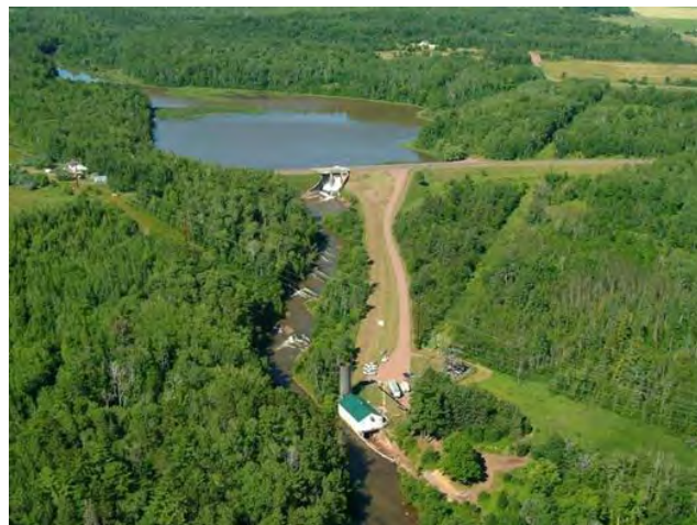
White River Dam
