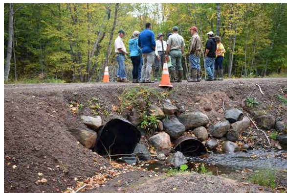
An interdisciplinary team of collaborators evaluates structural risk factors and FEH vulnerabilities at a road-stream crossing. Photo: WI Wetlands Association
