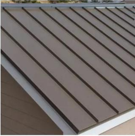
standing seam sheet metal roof
