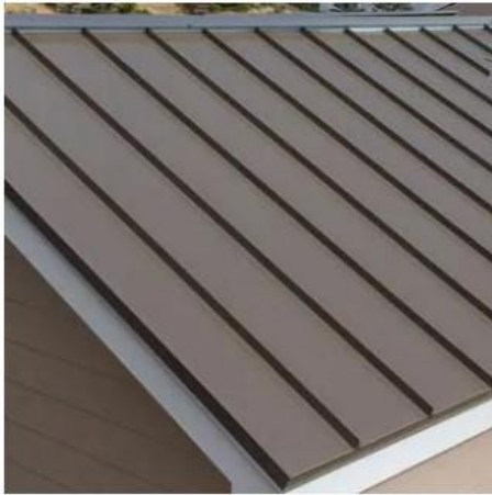
standing seam sheet metal roof
