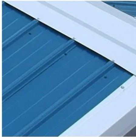
ribbed sheet metal roof
