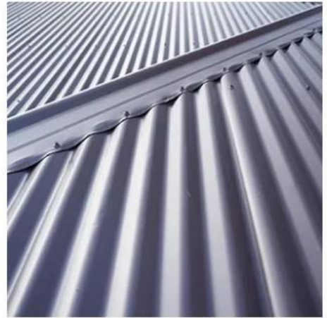
corrugated sheet metal roof
