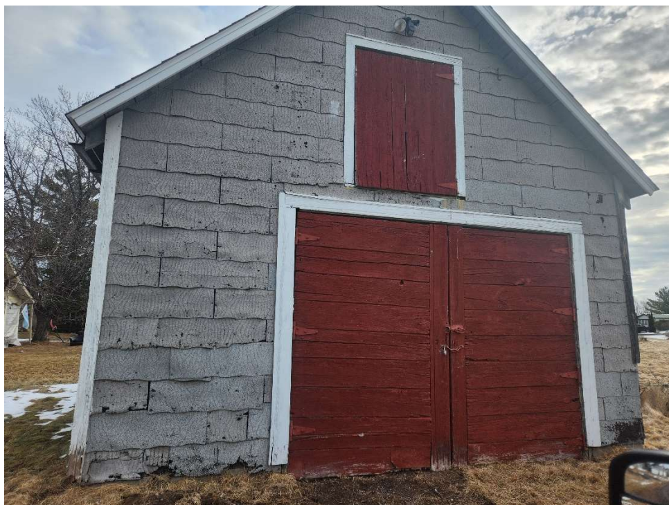
Front elevation of the existing shed
