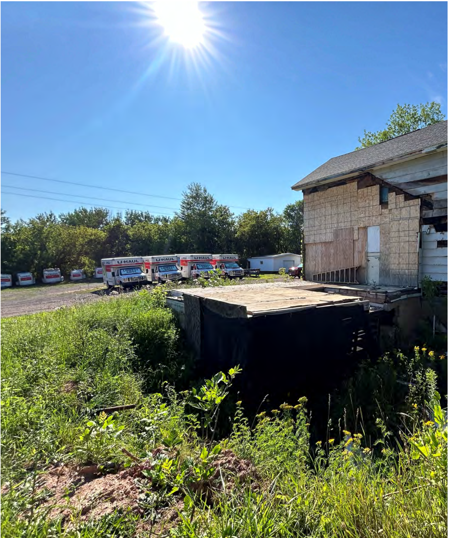
3. Permit #20240101 (relocated new garage on site): This project is approximately 95% complete now and looks nice on the property.
