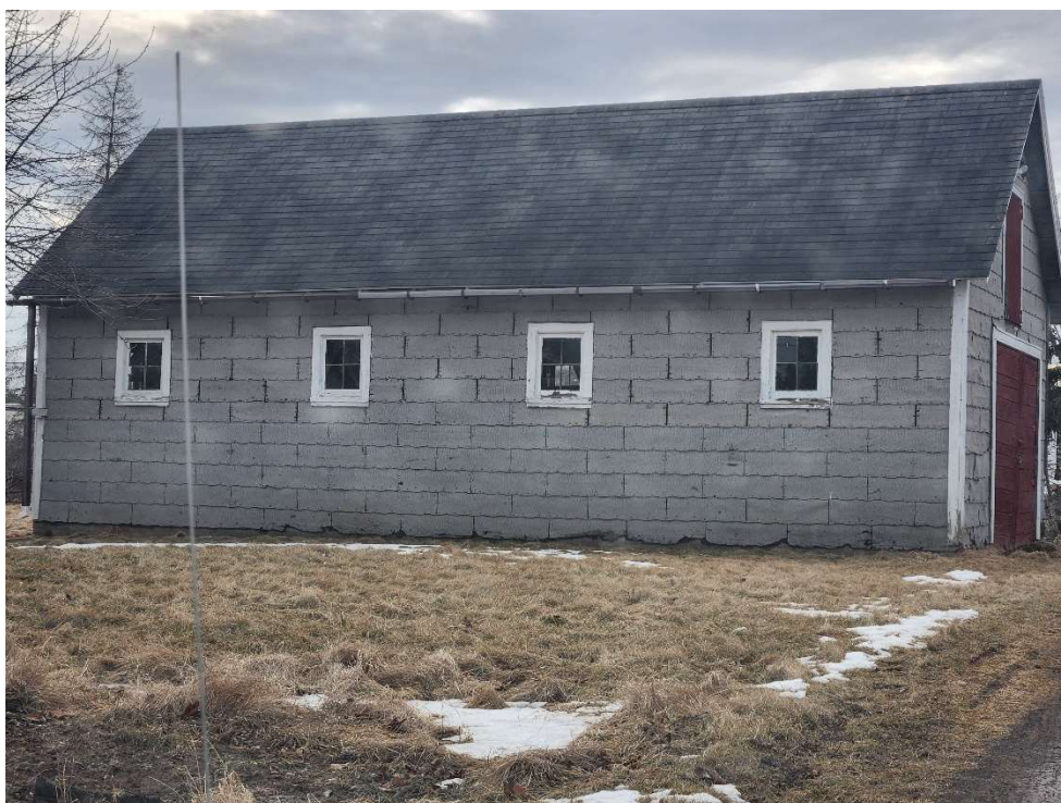
Side elevation of the existing shed
