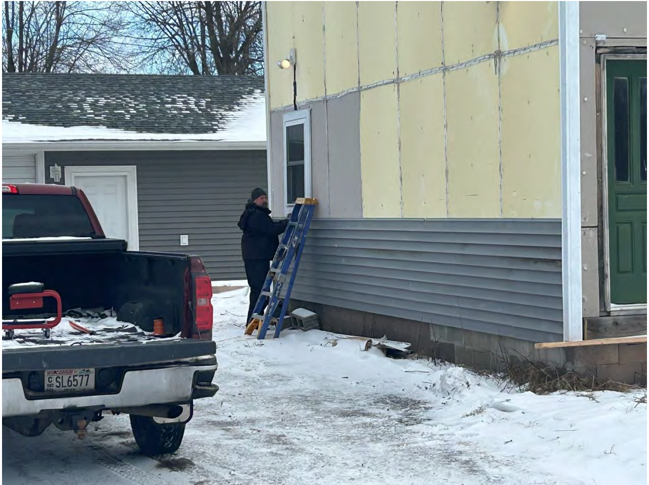
Photographs taken by Steve Schraufnagel on 01/16/2025 of Mr. Koenamann siding the house after the house was placarded and the placards removed
