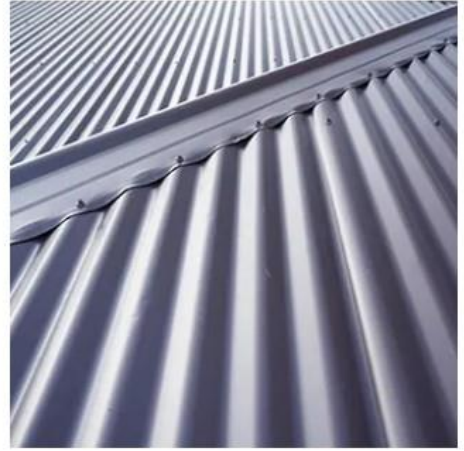
corrugated sheet metal roof
