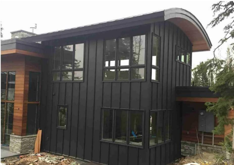
Painted standing seam metal panels with concealed fasteners. The finish is not shiny and the product looks
