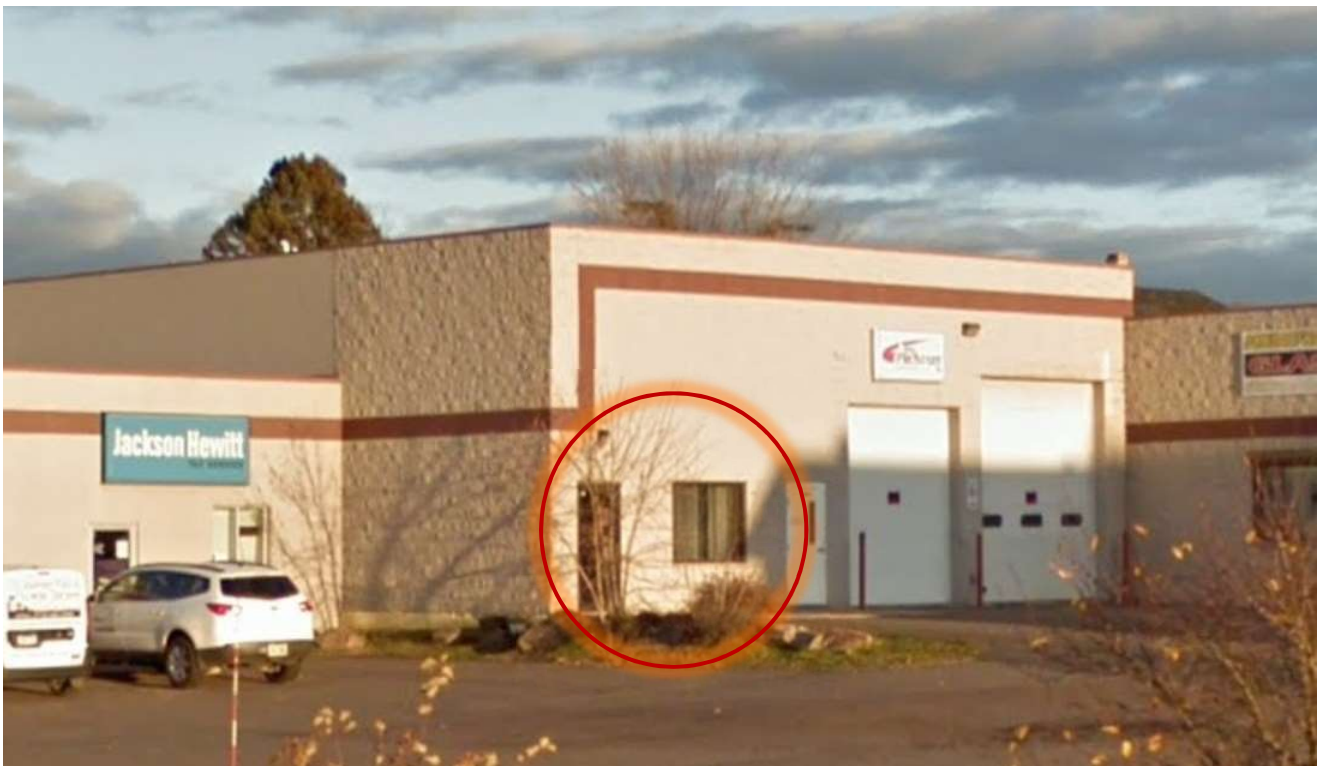
Photo looking at the main entrance to the office and the adjacent window
