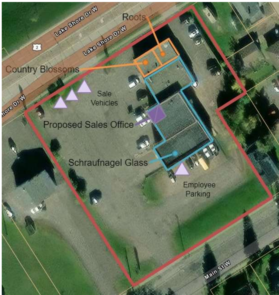
Enlarged Aerial View of Building and Parking Lot
