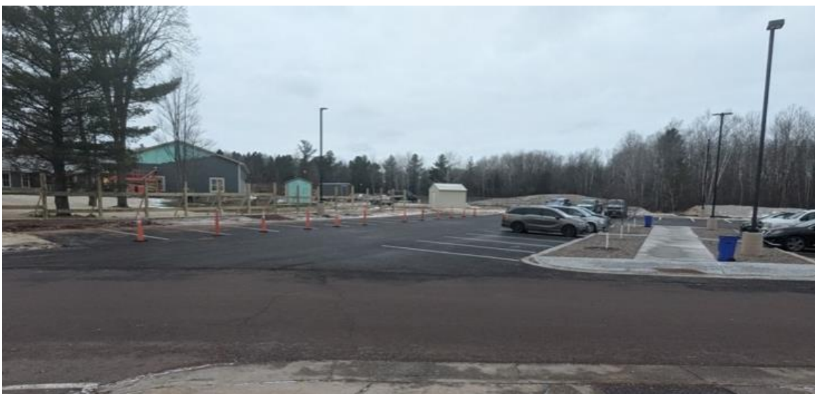
View from the South of the New Parking Lot Expansion and Behavioral Health Facility to the Left
