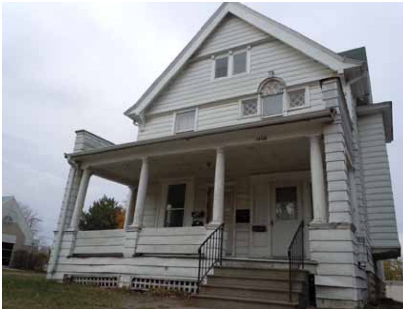
Figure 54: 1300 Third Avenue SE. Source: Web
