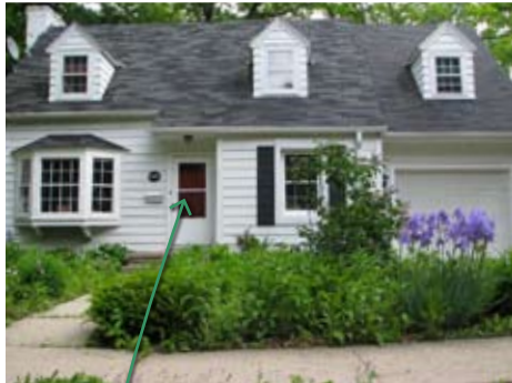
908 Talbot Ave. Colonial Revival
