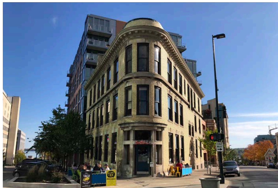
Jackman Building, 101 South Hamilton Street
