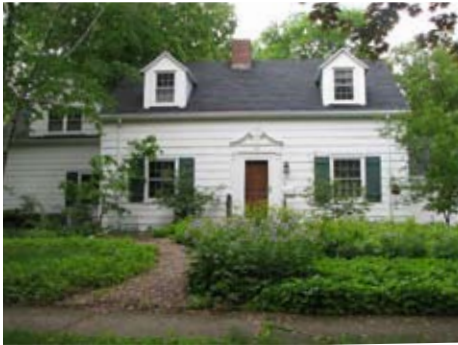
915 Talbot Ave Colonial Revival
