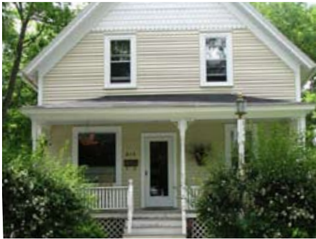
815 Oakdale Ave. Front Gable
