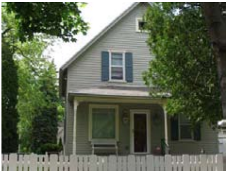
803 Oakdale Ave. Front Gable
