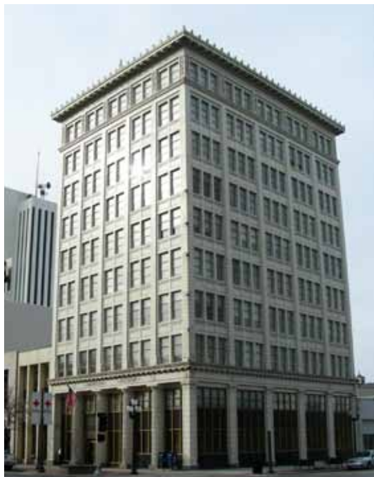
Figure 93: American Bank Building (1913-1914) at 101 Second Street SE.
