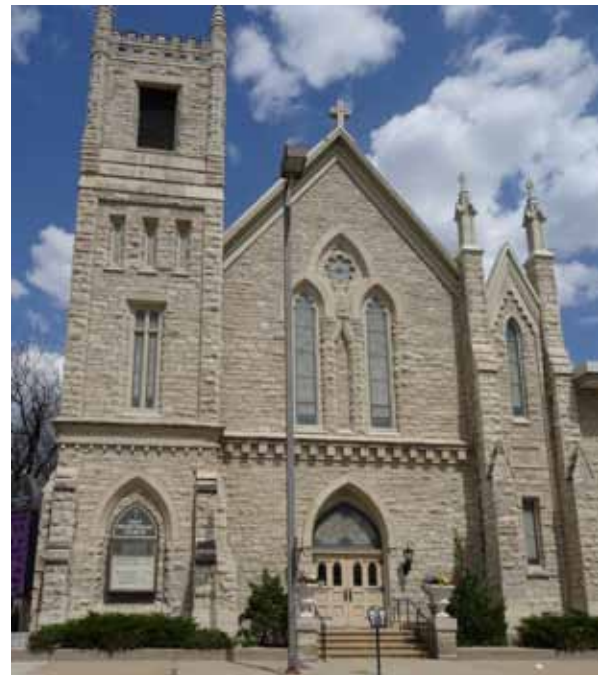
Figure 51: First Presbyterian Church (1869) at 310 Fifth Street SE.
