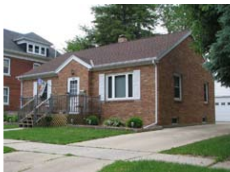
443 N. Superior St. Colonial Revival
