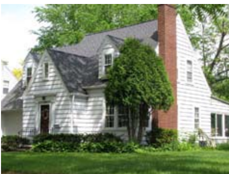
708 N. Michigan St. Colonial Revival
