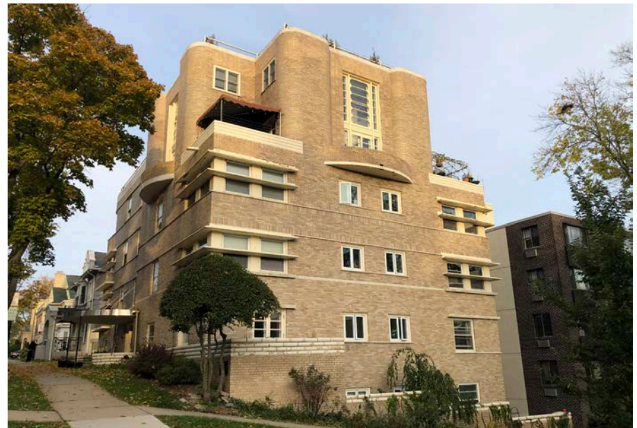
Quisling Towers Apartments, 1 East Gilman Street
