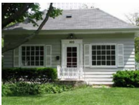
920 Oakdale Ave. One-story Cube
