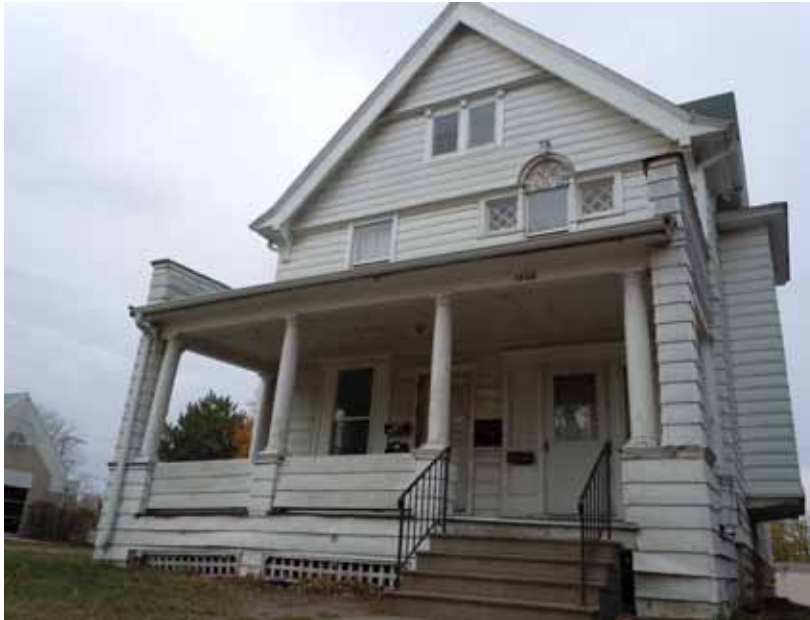
Figure 54: 1300 Third Avenue SE. Source: Web
