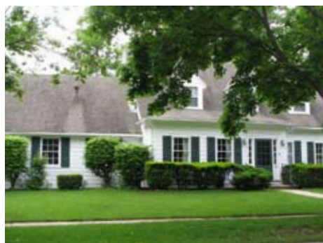
614 Randall Ave. Colonial Revival
