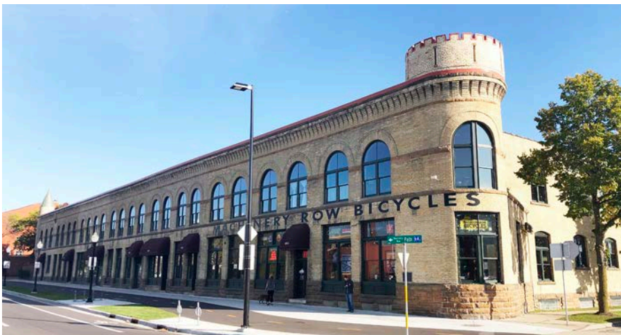
Machinery Row, 601-627 Williamson Street
