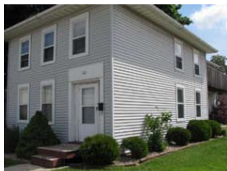
605 James St. Colonial Revival
