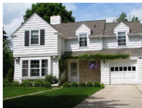
703 Ridgeway Blvd. Gable Ell
