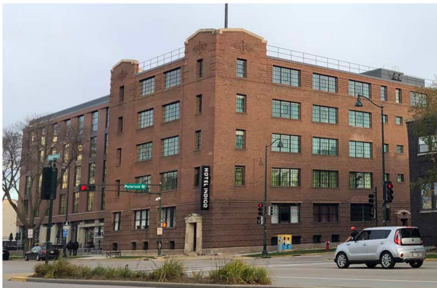
Klueter Wholesale Grocery Warehouse, 901 East Washington Avenue
