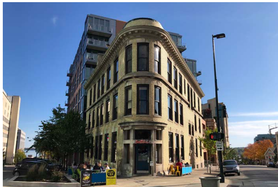
Jackman Building, 101 South Hamilton Street
