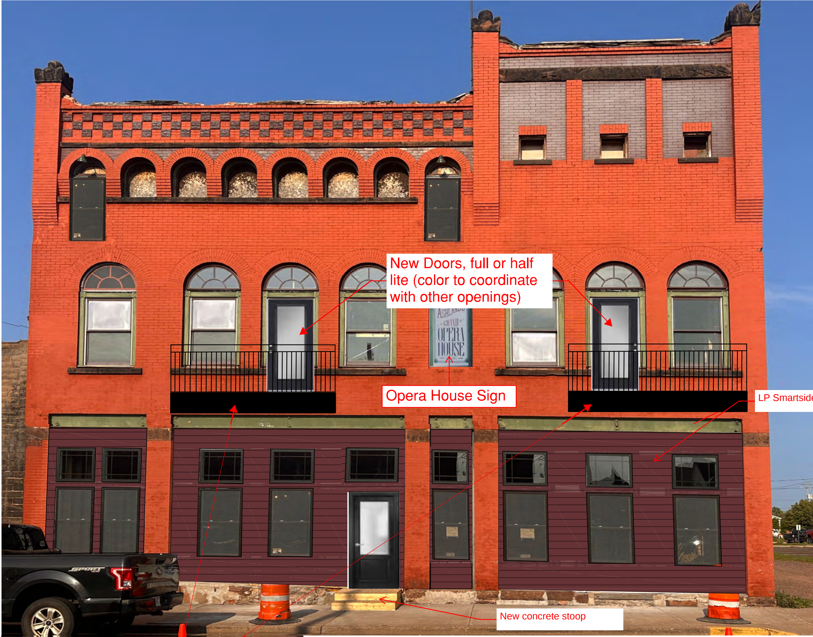
1 West Exterior Building Elevation 1/4" = 1'-0"
