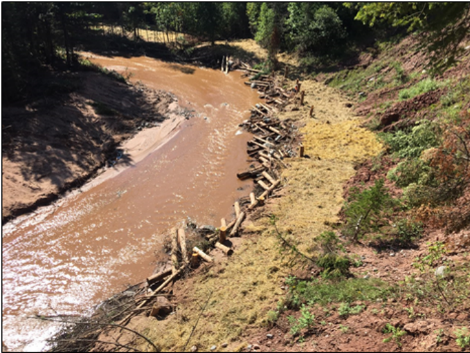
Figure 21: An Eroding Bluff On North Fish Creek Was Stabilized In 2018 Using A Log Cribwall. Similar Projects Are Recommended To Decrease The Sediment Load Of Chequamegon Bay.
