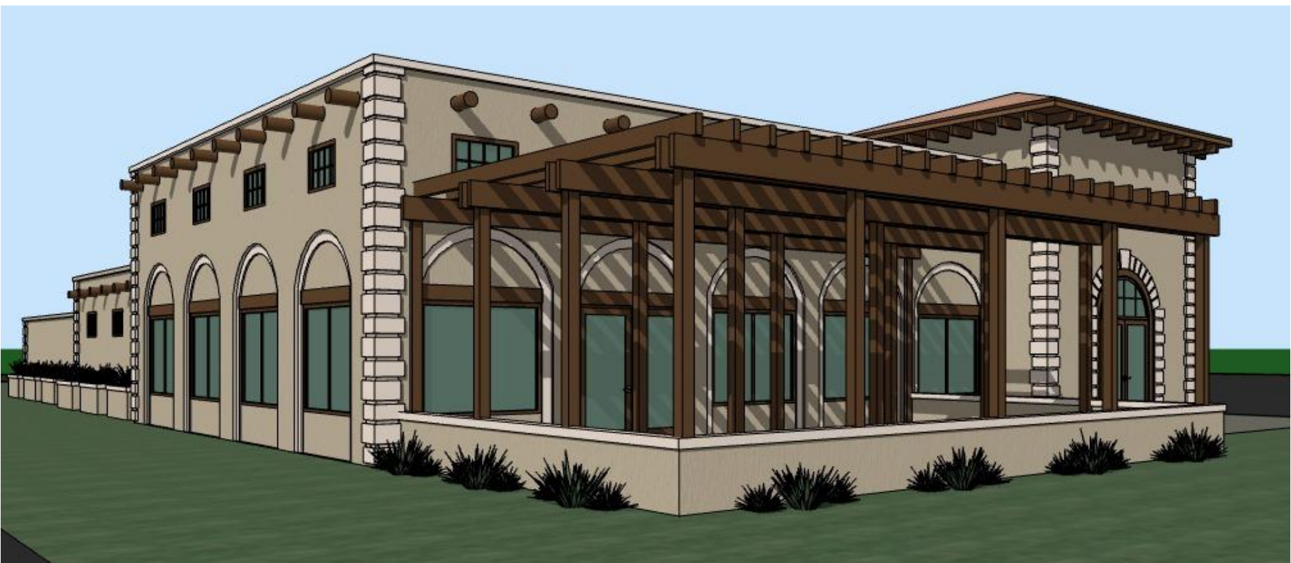
STREET VIEW (PATIO AREA)
