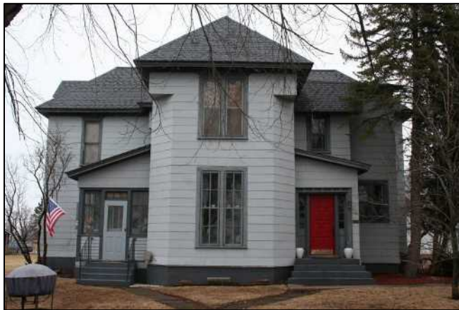
110 N. Ellis Avenue (aka 1 Fifield Place): Samuel S. & Stella Fifield House (1883).
