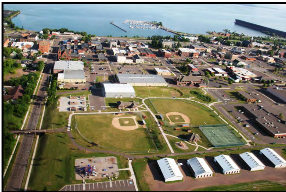
Central Railyard Park Complex: Major Community Park
