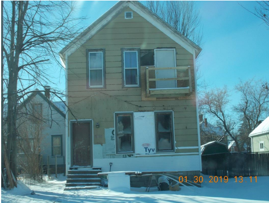
221 Stuntz Ave—Herschberger—5 (In process or residing/repairing)
