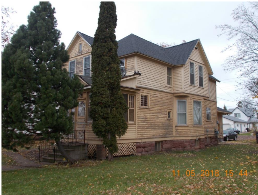
812 Vaughn Ave—MacIntyre—5 (Repaired roof with assistance through HIP in 2018, HIP will assist with paint and homeowner will be fixing foundation in 2019)
