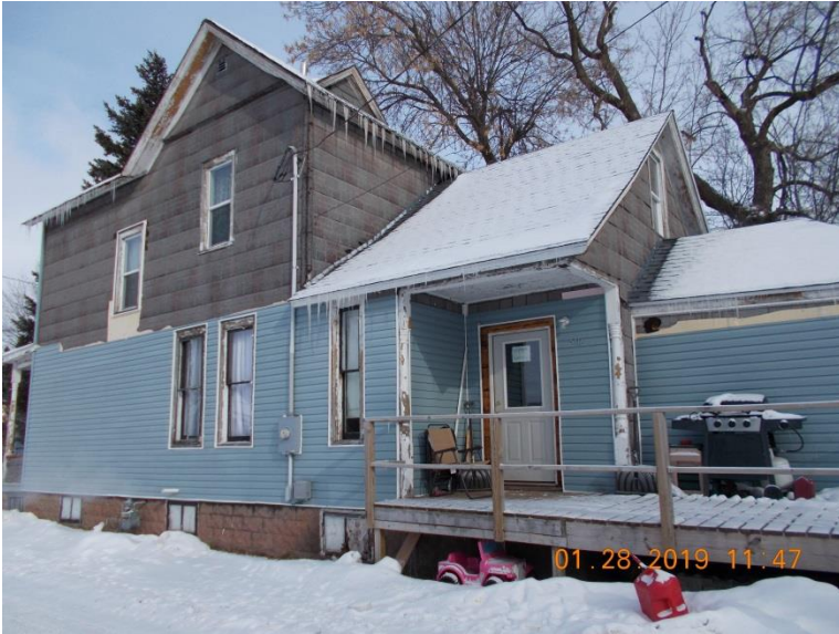
510 7 th St W—Zakovec—5+ (Siding in progress)
